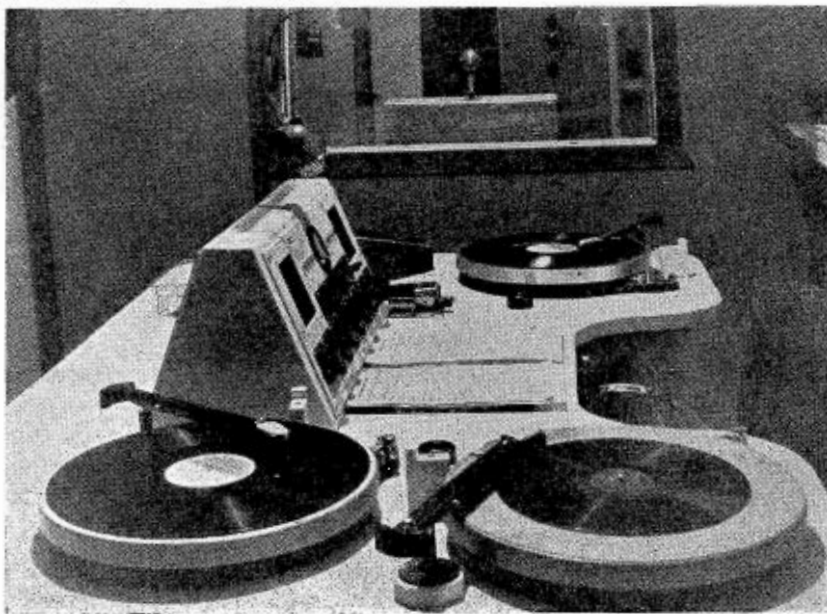
Recently Installed Announcing Control Table, 2MO.
