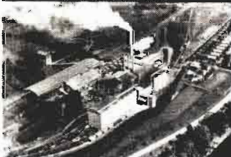
Lehigh Portland Cement, Allentown
