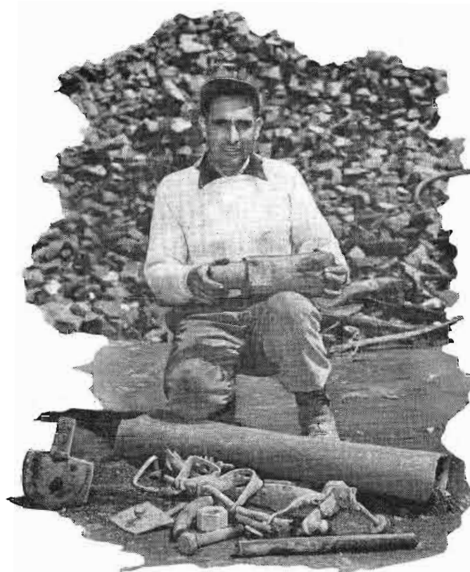
Workman displays some of the pieces of "tramp" metal which, if not spotted by RCA's metal detector, might have damaged rock crushing machinery.
