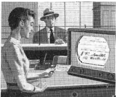
RCA vidicon camera in a bank, lets tellers verify the signatures on checks by television.
