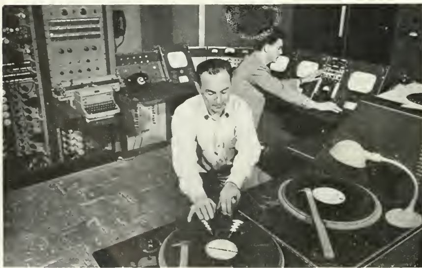
MASTER CONTROL ROOM OF TELEVISION STATION KRON-TV WITH VIDEO MONITORS IN REAR AND TRANSCRIPTION TURNTABLES IN FOREGROUND.
