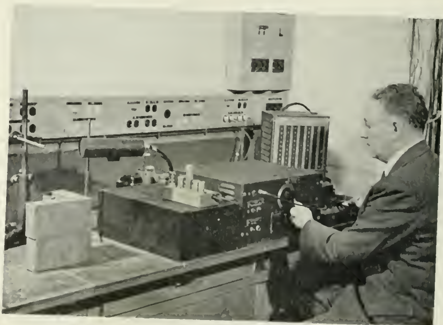
DR. G. A. MORTON OF RCA LABORATORIES SEATED BEFORE AN EXPERIMENTAL MODEL OF SCINTILLATION COUNTER EMBODYING A NEWLY DEVELOPED RCA MULTIPLIER PHOTOTUBE.
