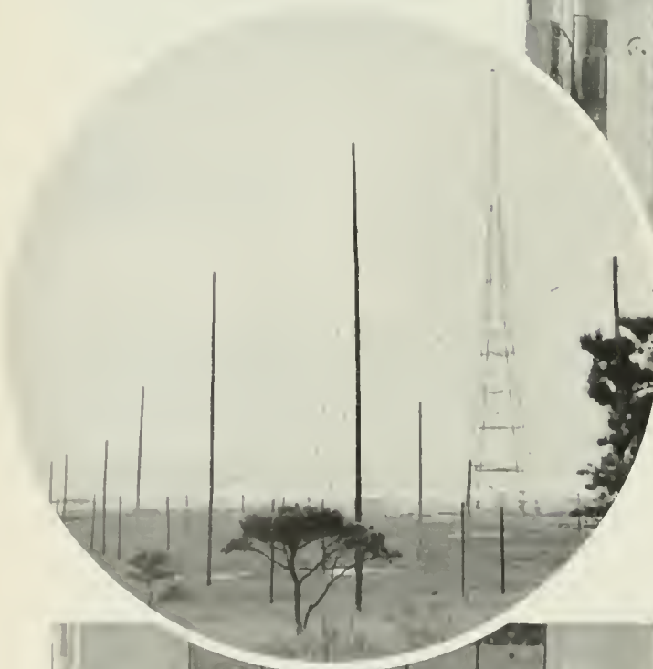
Beyond the lines of short masts supporting the station's high-frequency antennas is the high tower of Chatham's 500-kilocycle transmitter.
