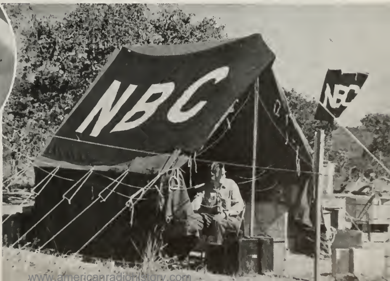
SIGNALS ORIGINATING IN THIS CANVAS-COVERED TRANSMITTER AT BOCAUYVA WERE SENT SOUTHWARD TO RIO DE JANEIRO AND THEN RELAYED TO NBC OVER A PROGRAM SERVICE CIRCUIT TO NEW YORK.
