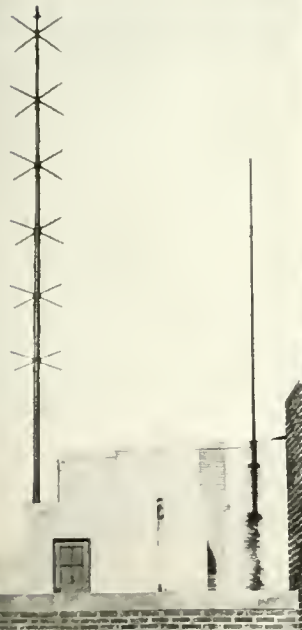
LEFT: FM "TURNSTILE" ANTENNA DEVELOPED BY RCA AND INSTALLED FOR A PHILADELPHIA STATION. CENTER: FIELD INTENSITY METER USED FOR MEASURING COVERAGE OF FM AND TELEVISION STATIONS. RIGHT: RADIO-TELEPHONE EQUIPMENT IN A POLICE CRUISING CAR.
