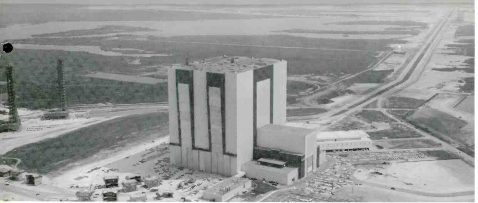
Saturn rockets will travel on launch umbilical towers (left) from Vehicle Assembly Building to launch pad over roadway at right.
