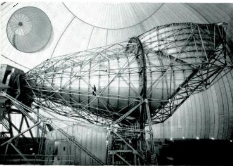
Giant horn antenna at the Andover, Maine, ground station.
