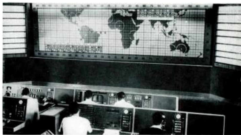
Far-ranging electronics system feeds data to Cape Canaveral.
