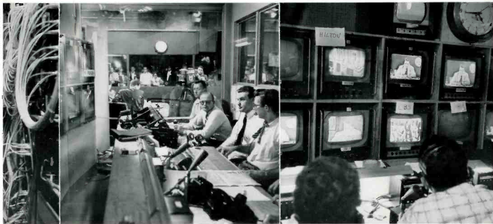
A technician trouble-shoots cables (above left) which carry the audio and video signals selected by Program Directors in the "On-The-Air" Control Room (above center) from the bank of TV monitors in front of them (above right).
