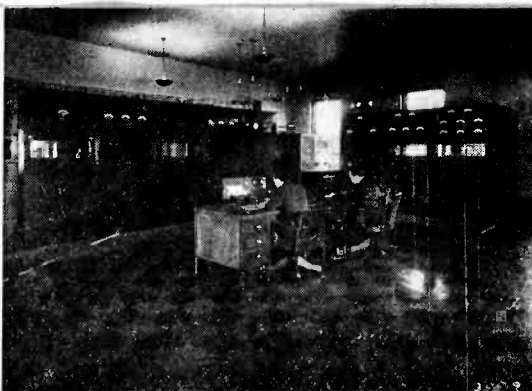
The main equipment room of WABC, showing the 50,000 watt transmitter and the 17,000 volt power supply. This station is located at Wayne, N. J., about 20 miles from New York City.
