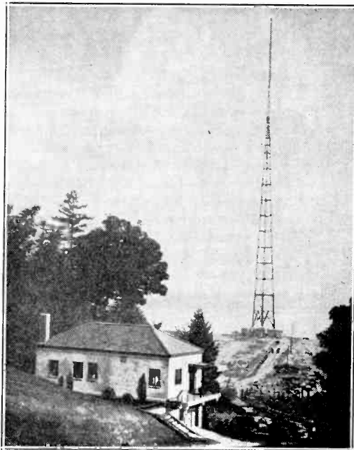
The new KVI aerial and transmitter house, on Vashon Island, Tacoma, Washington.
