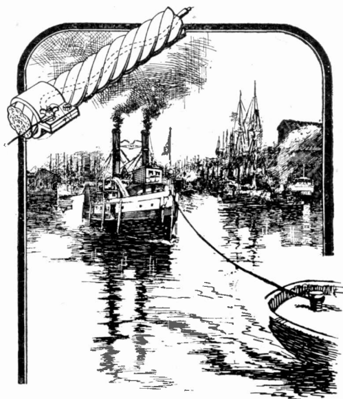
A TELEPHONE WIRE IS EMBEDDED IN THE TOW LINE
