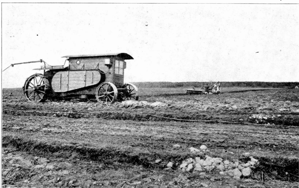
PORTABLE ELECTRIC GENERATING PLANT AS USED FOR PLOWING IN GERMANY
