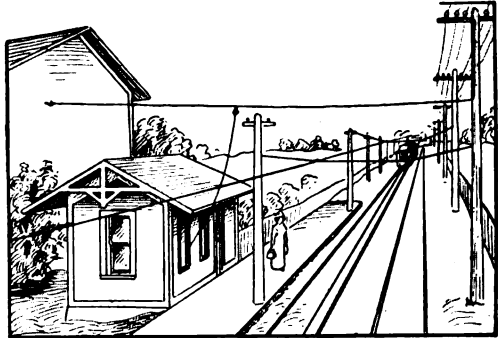
Fig. 1. Running Bridle Wire Over Trolley Line
