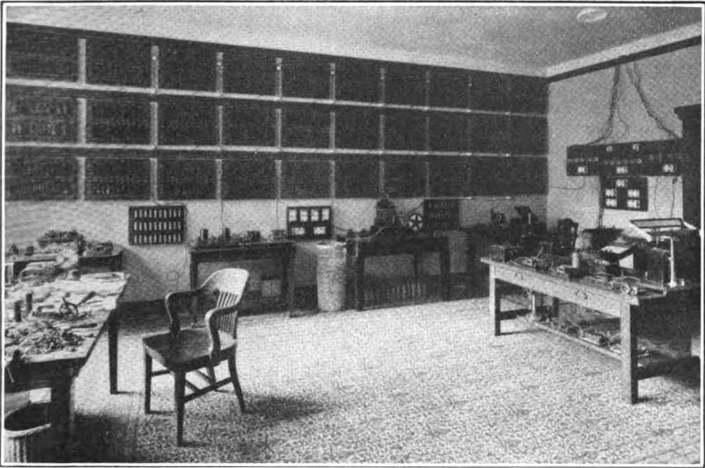
The Bank of Resistances and Capacities at the Farther Wall Represents, Electrically Speaking, Several Thousand Miles of Ocean Cables
