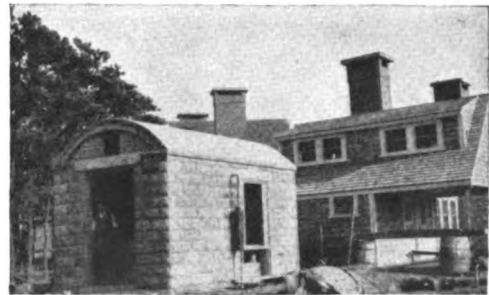
Powerhouse with Main Office in Distance
