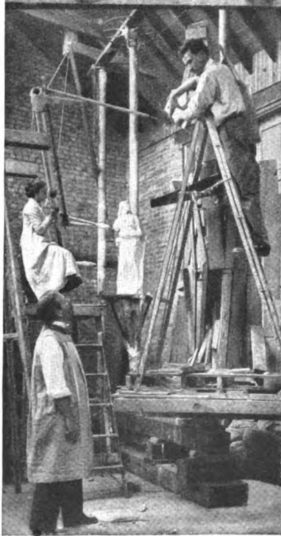
Mr. Taft Superintending the Construction of the Framework for a Large Statue
