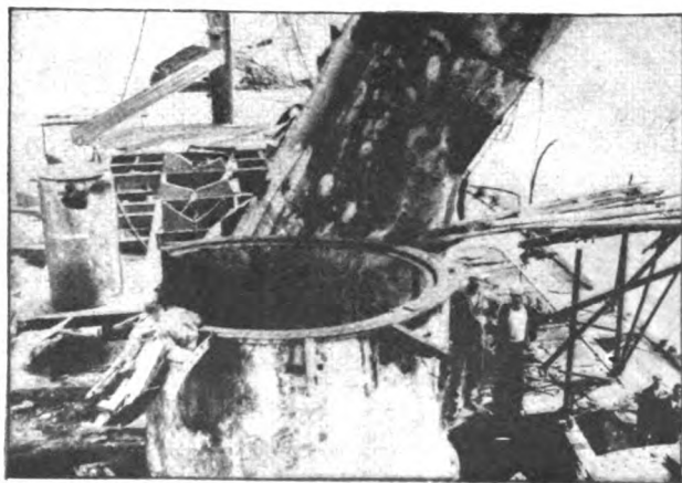
The Basket Work or Cage Mast Is Essentially an Institution in the American Navy; Other Navies the World Over Have Pronounced It Valueless. The Mast Shown in the Photograph Was Erected on the San Marcos and Made the Target of the Idaho. It Took More than a Dozen Shots to Bring the Fire Control Mast Tumbling Down. One Shot Wrecked the Old Style "Fighting Top" Mast
