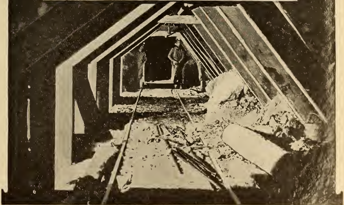
THE ELEMENT OF DANGER—MANY OF THE TUNNELS MUST BE HEAVILY TIMBERED
