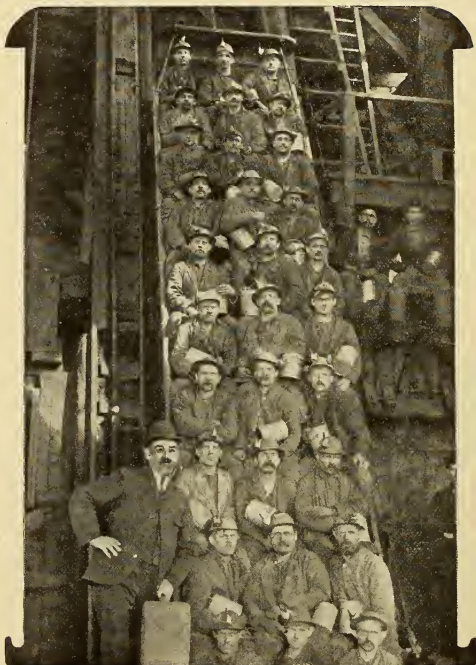
LOADED MAN-CAR READY FOR THE MILE PLUNGE INTO THE EARTH. IF THE CABLE SHOULD BREAK, THE CAR WOULD STRIKE THE BOTTOM TRAVELING AT THE RATE OF OVER FOUR MILES A MINUTE
