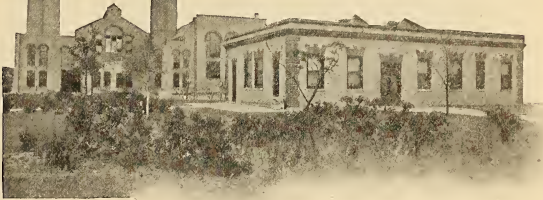
ATHLETIC FIELD AT HAWTHORNE AND THE GREAT POWER HOUSE THAT SUPPLIES THE WORKS
