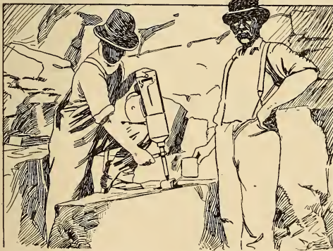
THE PLUG DRILL WILL MAKE A HOLE FOUR INCHES DEEP AND ONE INCH IN DIAMETER IN ABOUT THREE MINUTES
