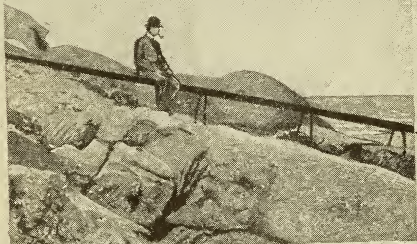
CABLE CONNECTING THE BELL TO THE POWER PLANT
