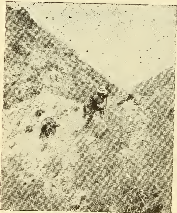
Digging pole holes in the rocky hillside
