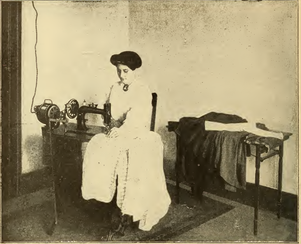
UTILITY MOTOR ATTACHED TO SEWING MACHINE
