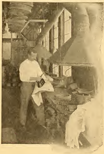
A FEW DEFT PASSES OF THE "HAND SHELL" FLANGE AND CURL THE BRIM
