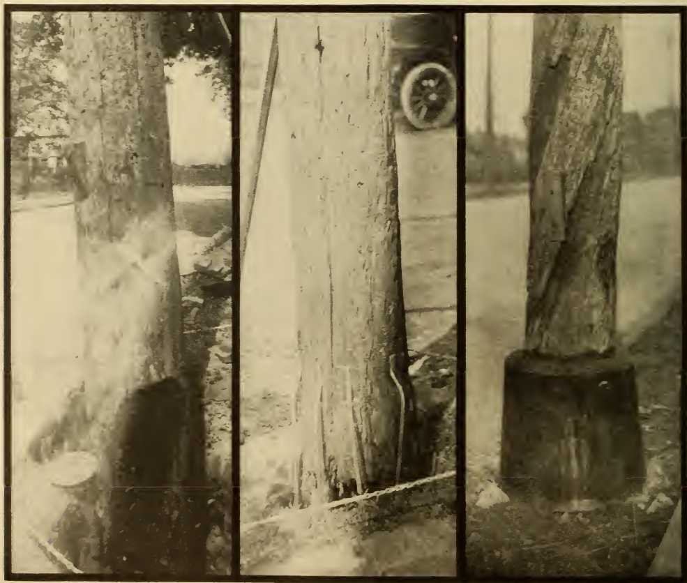
STEPS IN THE METHOD OF POLE REINFORCEMENT
