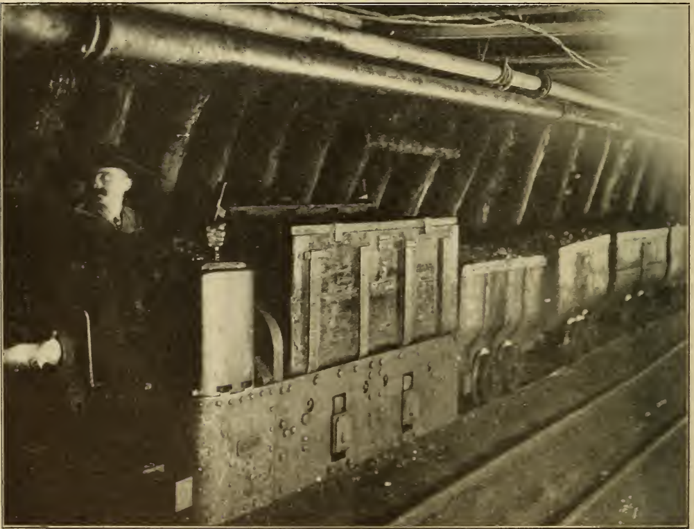
FIG. 1. STORAGE BATTERY LOCOMOTIVE IN THE MONOPOL MINE
