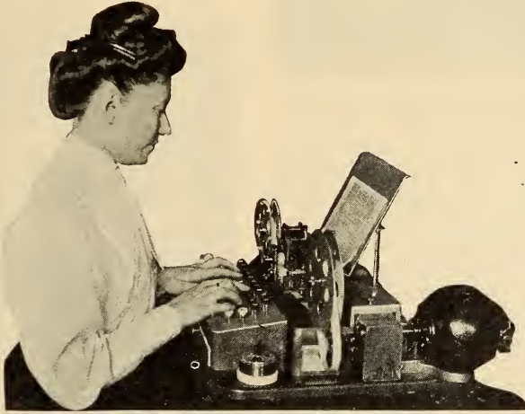
PERFORATING THE SENDING TAPE
