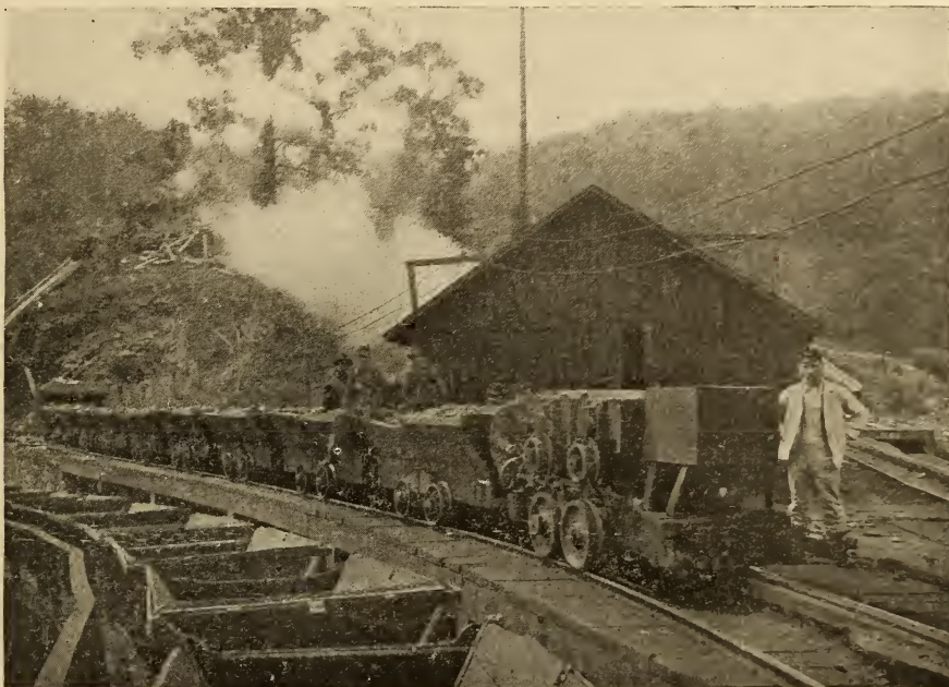
MINE LOCOMOTIVE AND A TRIP OF LOADS.
