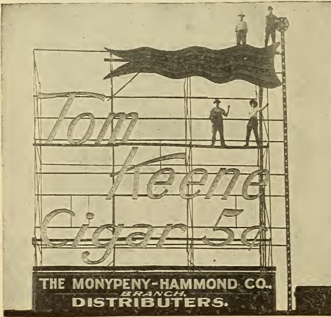
FIG. 3. WAVING FLAG EFFECT FROM TWO-PART COMBINATION FLASHER.
