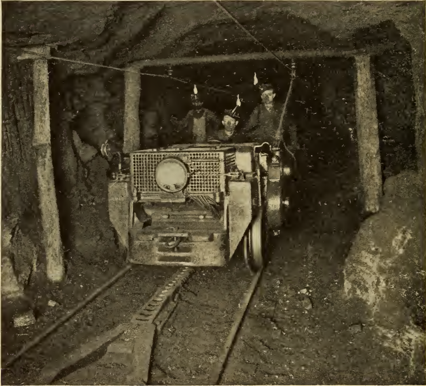
MINE LOCOMOTIVE AT THE END OF A TRACK SECTION.
