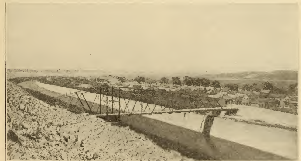
VIEW ON THE DRAINAGE CANAL.
