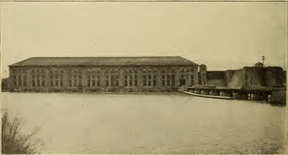
EXTERIOR OF CANAL POWER HOUSE.
