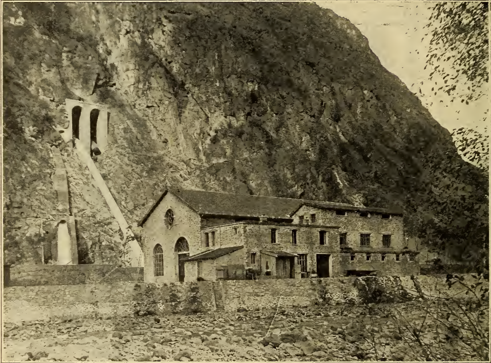
SCHILIENE WATER POWER ELECTRIC PLANT.
