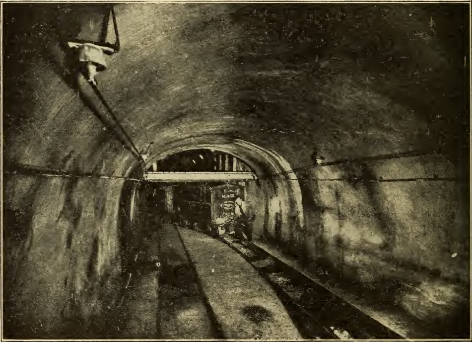
CHICAGO FREIGHT TUNNELS.
