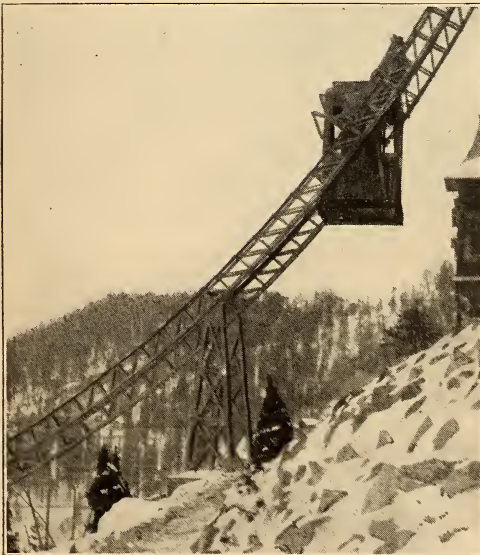
ELECTRIC ELEVATOR ON MOUNTAIN SIDE.
