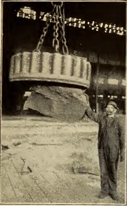
FIG. 1. LIFTING MAGNET RAISING 5,500-POUND "SKULL" OF IRON.
