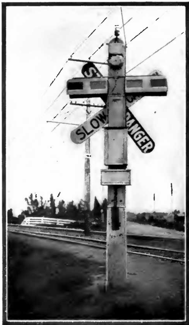
A New Type of Railroad Crossing Signal in which the Arms Change Position to Warn Oncoming Pedestrians and Drivers.
