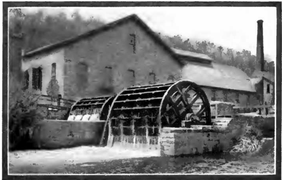
An Ingenious Water Wheel Arrangement in Which the Power is Applied to Another Wheel in Order to Raise Water to a Higher Level.
