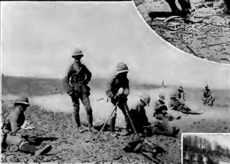
An Example of the Ingenuity of French Soldiers. The Cylindrical Frames Made of Wooden Sticks and Twisted Twigs are Filled with Earth and Used to Cover the Guns When They are not in Action.
