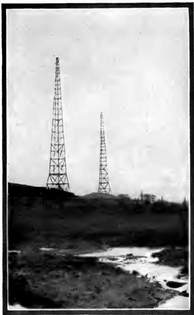
The Steel Towers of the Aerial of the Chelsea Station, and the Wireless Station Building.
