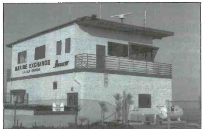
Vessel traffic system command center, overlooking harbor entrance.
