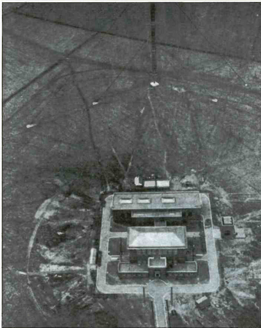
Station 5XX, the BBC's magnificent 26 kW longwave broadcast station at Daventry. This 1926 view was from the top of one of its two towers. The other tower is at the top of the photo.
