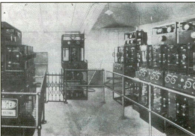
The 3 kW transmitter used by 2LO. It was installed on the roof of Selfridge's, London.
