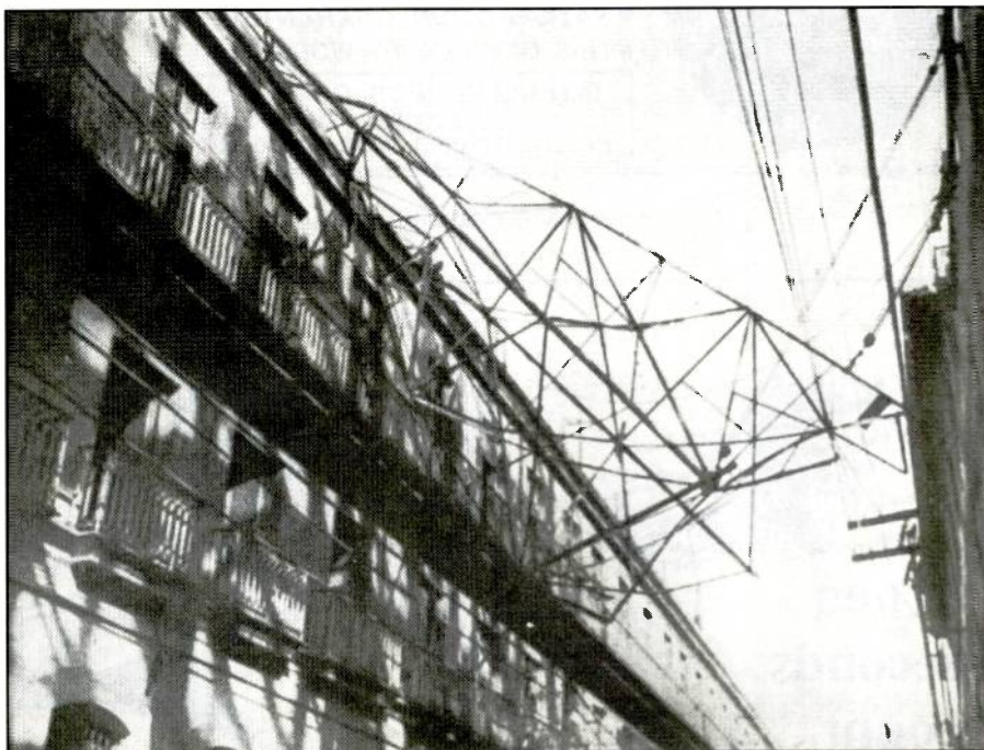
In 1927, a hurricane knocked the PWX antennas off the roof of the Cuban Telephone Building.
