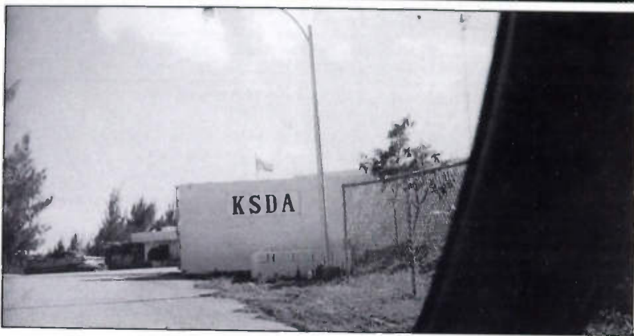
Here's the transmitter building of KSDA on Guam. (Thanks to "Bug Hunter")
