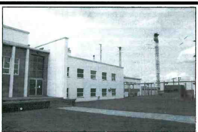
This view is of the RCI Sackville transmitter building. Thanks to Gary Hubert of Ontario.
