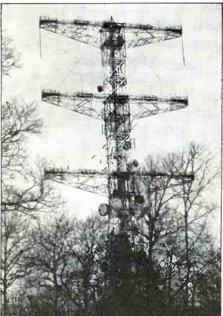
A 1991 look at the wonderful FM transmission tower built more than 50 years ago by Major Armstrong at Alpine, NJ. Today it is home to many repeater and microwave antennas. (Photo by Mark J. Rosen, NY.)
