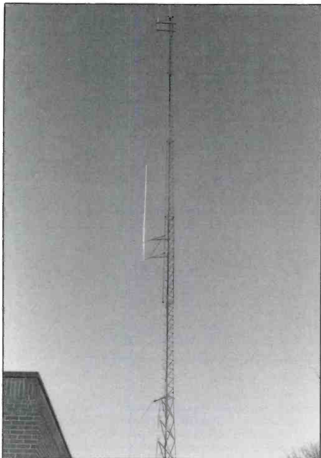
The State of Illinois Emergency Services and Disaster Agency base station tower, Marion, IL. This tower supports antennas for low/high band VHF, also UHF.
