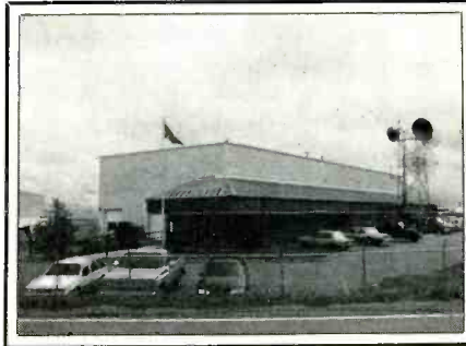
The U.S. Forest Service Rocky Mountain Region Aviation and Fire Service Center dispatches a five-state region from this building at the Jefferson County Airport north of Denver.
