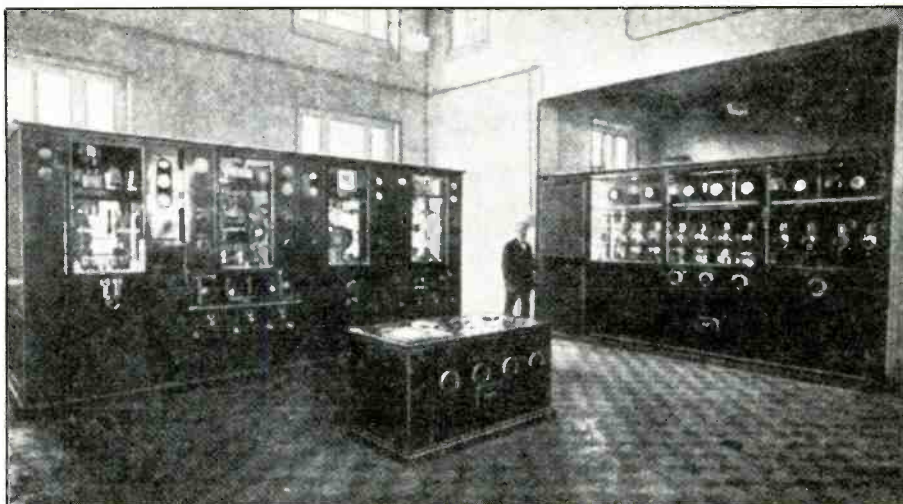
One of the Radio Colonial transmitter rooms at Pontoise.
