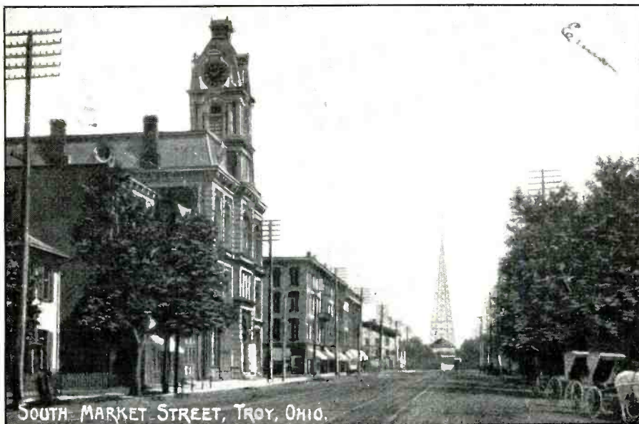
The Troy, OH mystery tower as it looked as seen from South Market Street.
