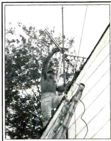
An existing and unused mast was selected.
