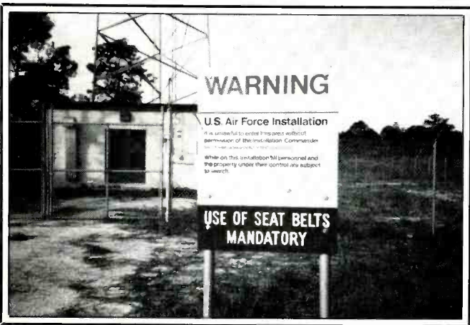
One of the (possible) HF towers at the tracking station.
