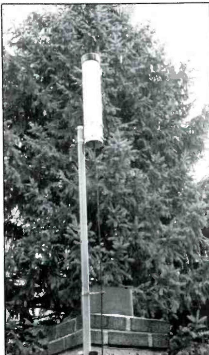
Fig. 1. Outdoor mounting of Dressler ARA500 active antenna.
