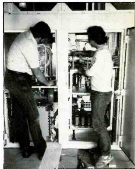
KUSW engineers Rex Carlson (1) and Ken Meyer.
