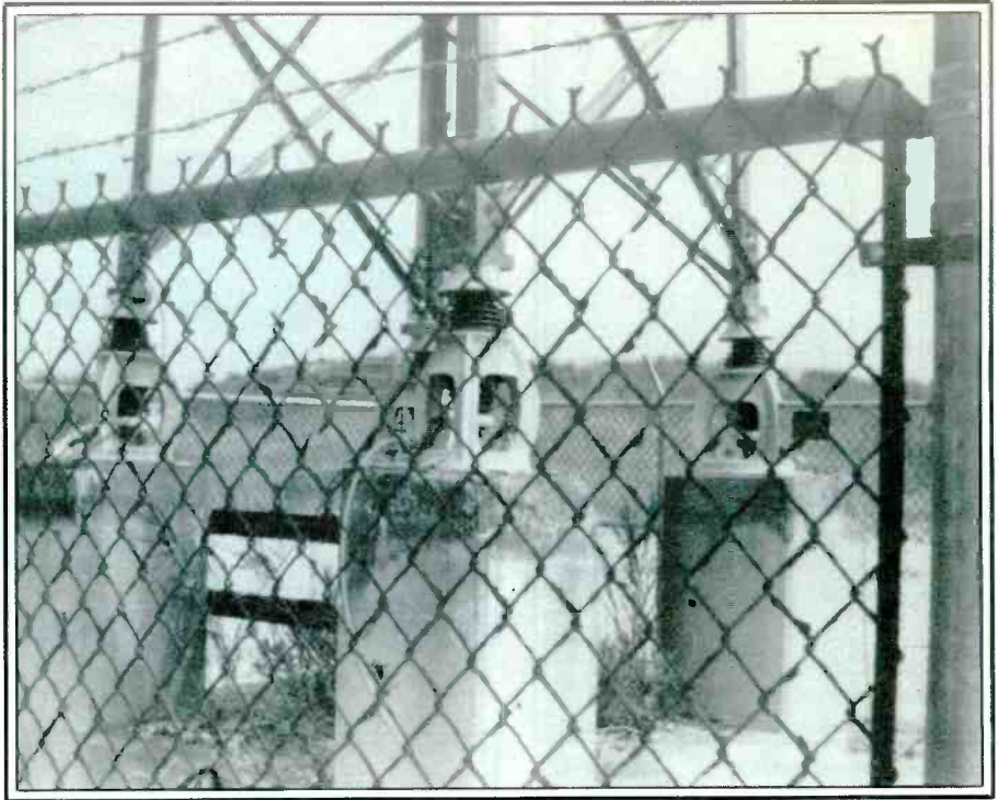
A close view of the insulated base of the Fire Island abandoned radio tower looks too modern to date back to 1918.
