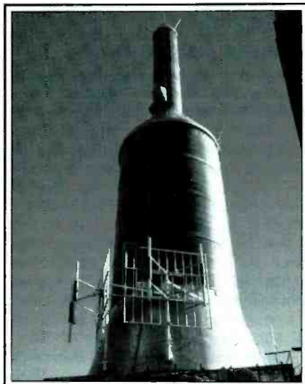
This isn't a Saturn rocket. It's the TV transmitter located 12,750 feet atop Mt. Blanc. A protective dome assembly with VHF link antennas are mounted near its base. (All photos by Lance McGraw)
