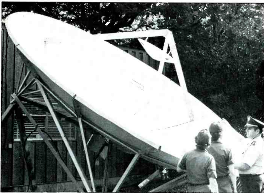
Programs are sent from the Army's Academy of Health Sciences via this transmitting dish, which feeds them into the WESTAR III satellite. Downlink frequency is 4160 MHz. (U.S. Army photo)
