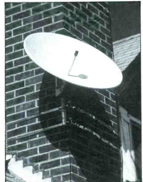
DBS rooftop dish installation. Photo courtesy of STC (Satellite TV Corporation).
