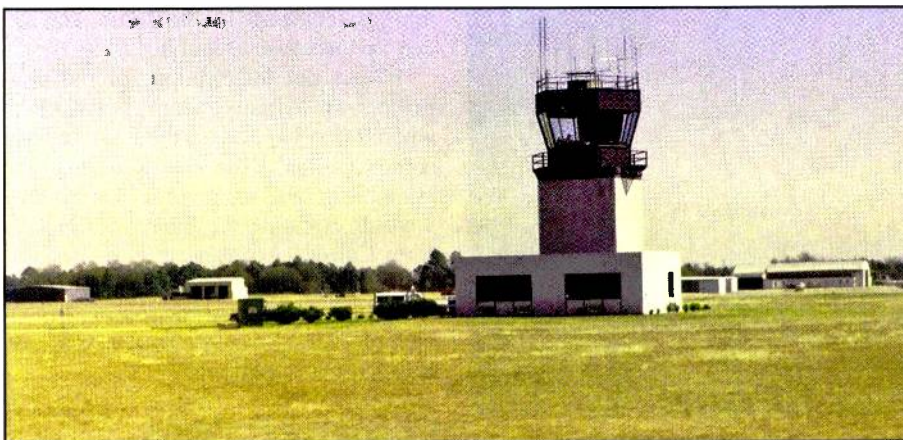
From the ground, here's the Albany (KABY) control tower — appearing as that little speck viewed from the sky in the picture above.
