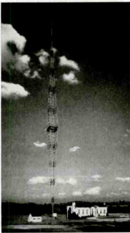
323 Feet Higher Than The Washington Monument
