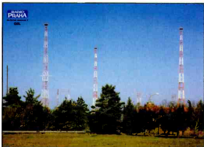
Radio Prague's former towers at the Litomyšl transmitter site.
