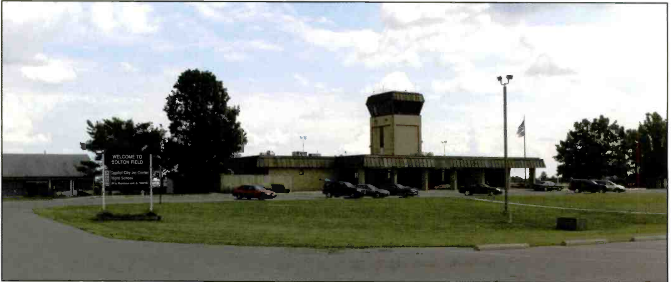
The tower and small terminal building at Bolton Field, Columbus, Ohio. The tower is only open part time. (Photo by Tom Swisher ©2010)
