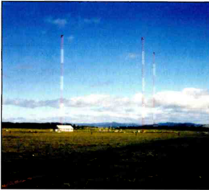
The Radio New Zealand International transmitting towers at Rangataiki.
