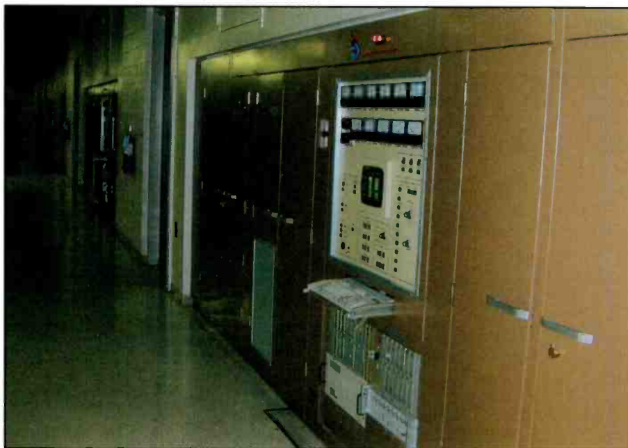
A new 500-kW transmitter at WEWN, currently running at 250. (Thanks Charles Maxant)
