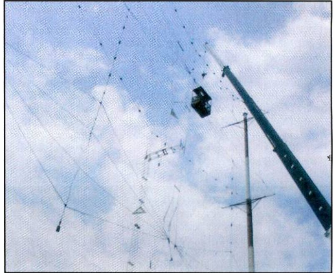
Damaged antennas under repair at WMLK, Bethel, Pennsylvania. (Thanks Charles Maxant, WV)
