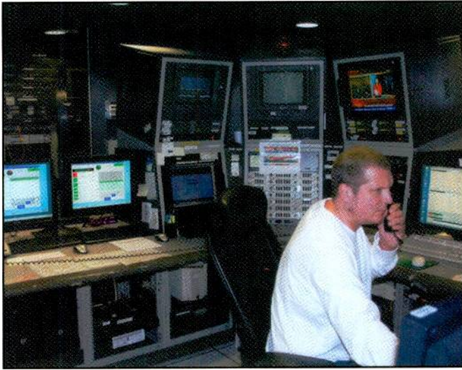
Computers control much of what goes out on RFA transmitters.
