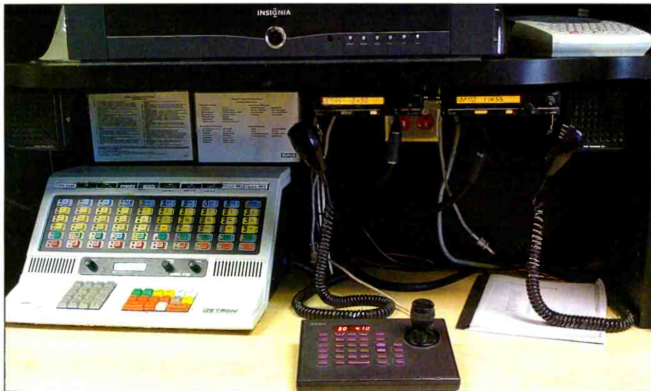
The Snow Operations Desk at an international airport. The console on the left is used for access to airport operations channels, while the two ICOM aviation radios mounted under the shelf are used for monitoring Tower, Ground, and De-Icing frequencies.
