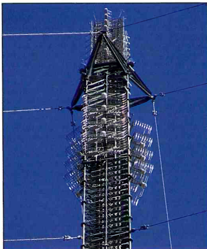
Photo C. In the top section you see is the circular polarized broadcast antennas for the six combined transmitters (see text).
