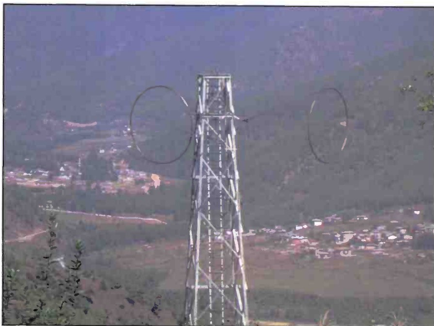
BBS' new shortwave antenna for its 100-kW transmitter is helping expand the station's reach. (Photo by Thinley Dorji, junior engineer, BBS)
