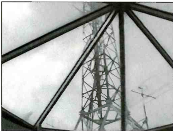
Through REE's skylight one can see the transmission tower linking the studio to the Noblejas transmitter site.
