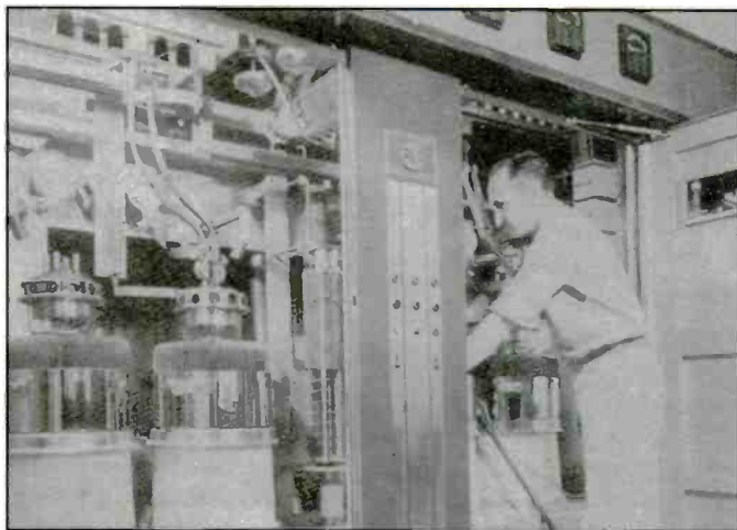
To the left of the WGAR transmitter engineer is a pair of power amplifier tubes. Each weighs over 350 pounds! This shot was probably snapped during the June 1947 installation of the Cleveland station's new RCA equipment. Besides the fact that interlocks would immediately shut down the transmitter if anyone opened the doors while it was running, the engineer's casual expression gives experienced RF folk the distinct impression that the picture was posed without any current flowing through the rig.
