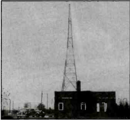
A 384-foot Truscon brand self-supporting tower watches over WGAR's 1000 Harvard Avenue transmitter building. The snapshot is probably from late 1935 or early 1936.
