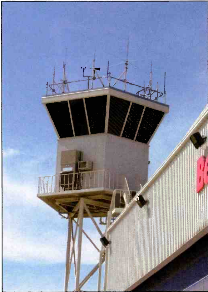
Note the many antennas on the Bell MV-22 tower used to communicate with MV-22s on test flights. (Photo by Steve Douglass)
