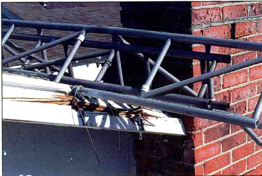
If you use your home's fascia as a tower brace, it's best to reinforce it so it won't split like this one did!
