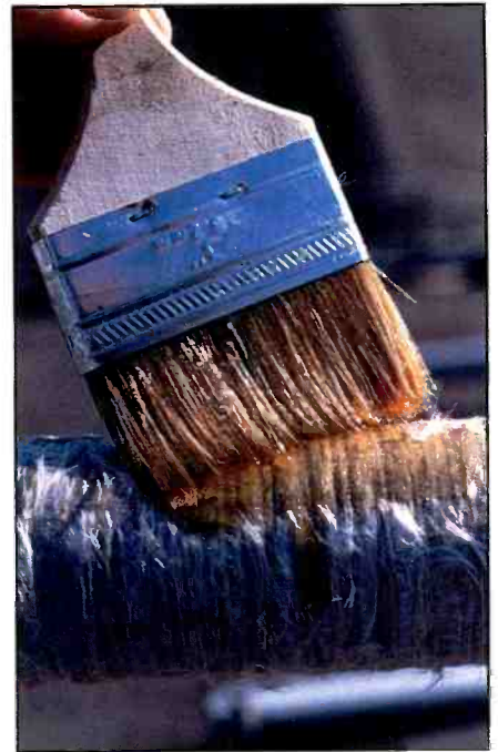
Brush on a clear coating of fiberglass repair resin to reseal your commercial antennas.
